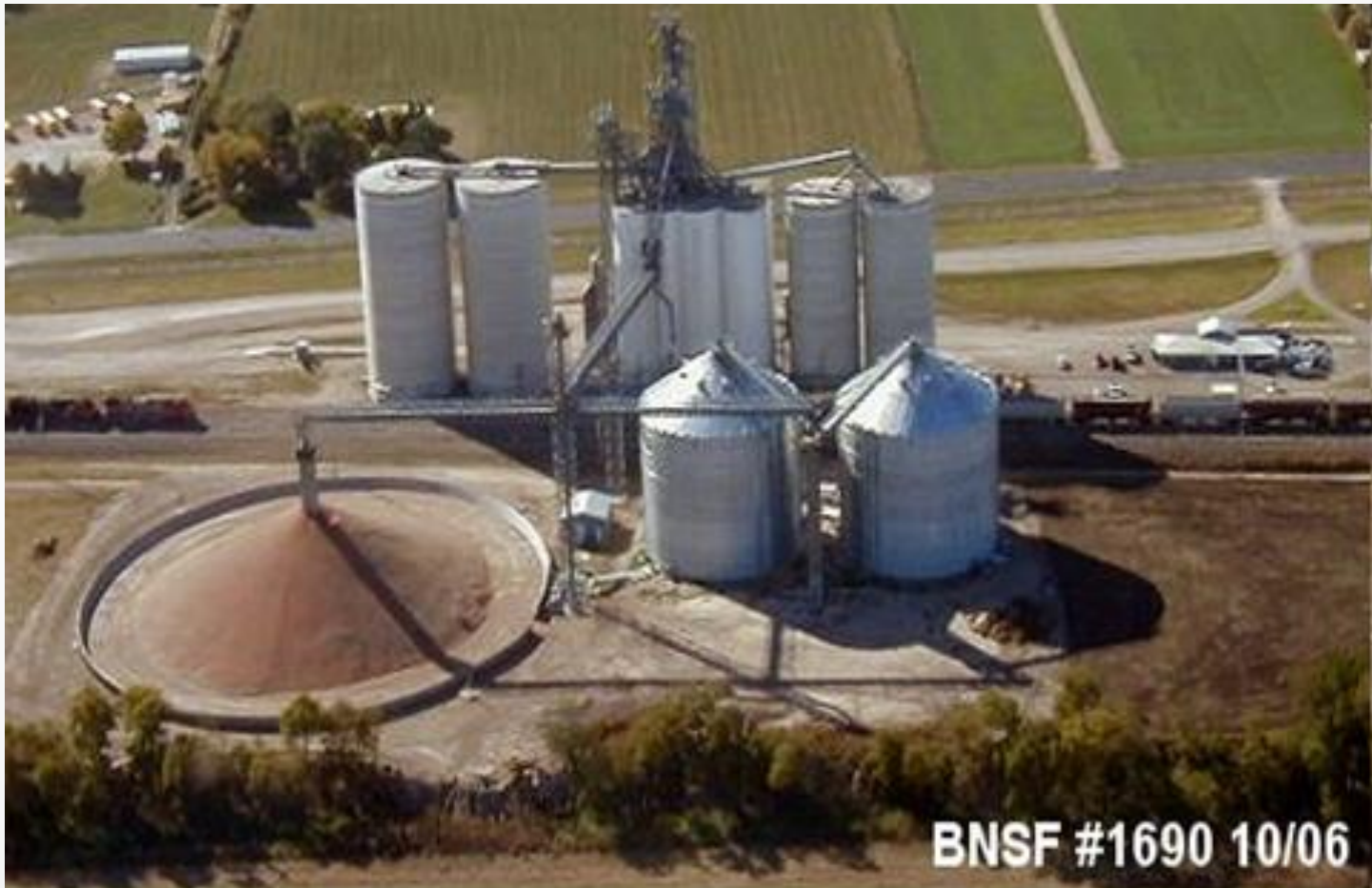
AgMark Co-Op Concordia, KS 4.75 million Bushels = 120,656 mt storage capacity
