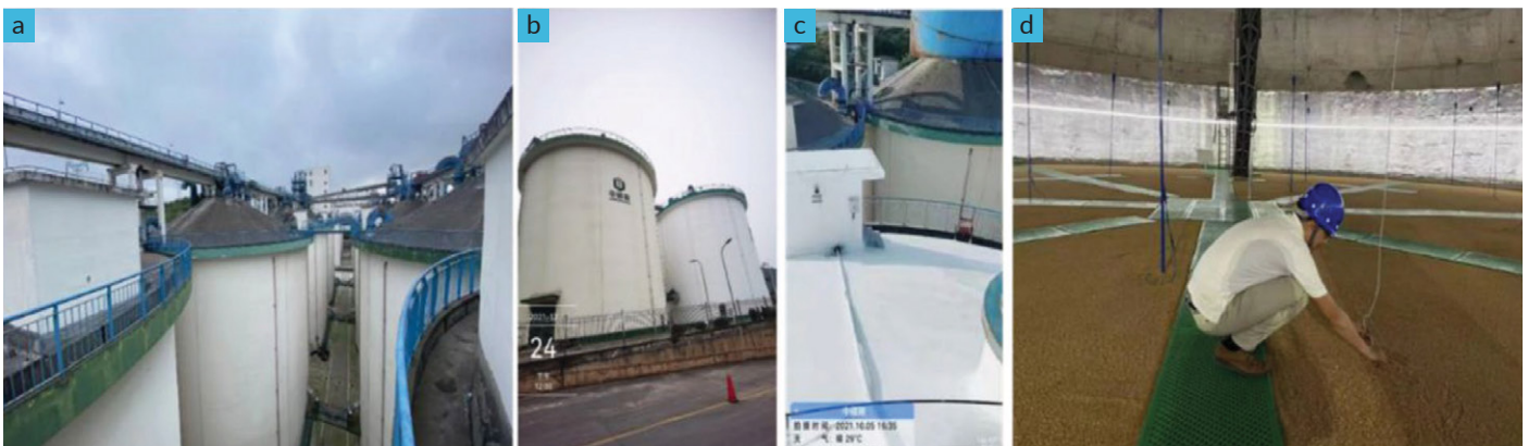
Typical grain silos in Chongqing Municipality, China. (a) Overhead view of the silos without the SSC-PSDRC coating; (b) groundview of the silos with and without the SSC-PSDRC coating; (c) bird's-eye view of the partial roof surface painted with the SSC-PSDRC coating; (d) interior view of the silo while installing the thermistor to measure interior temperatures of the wheat piles.
