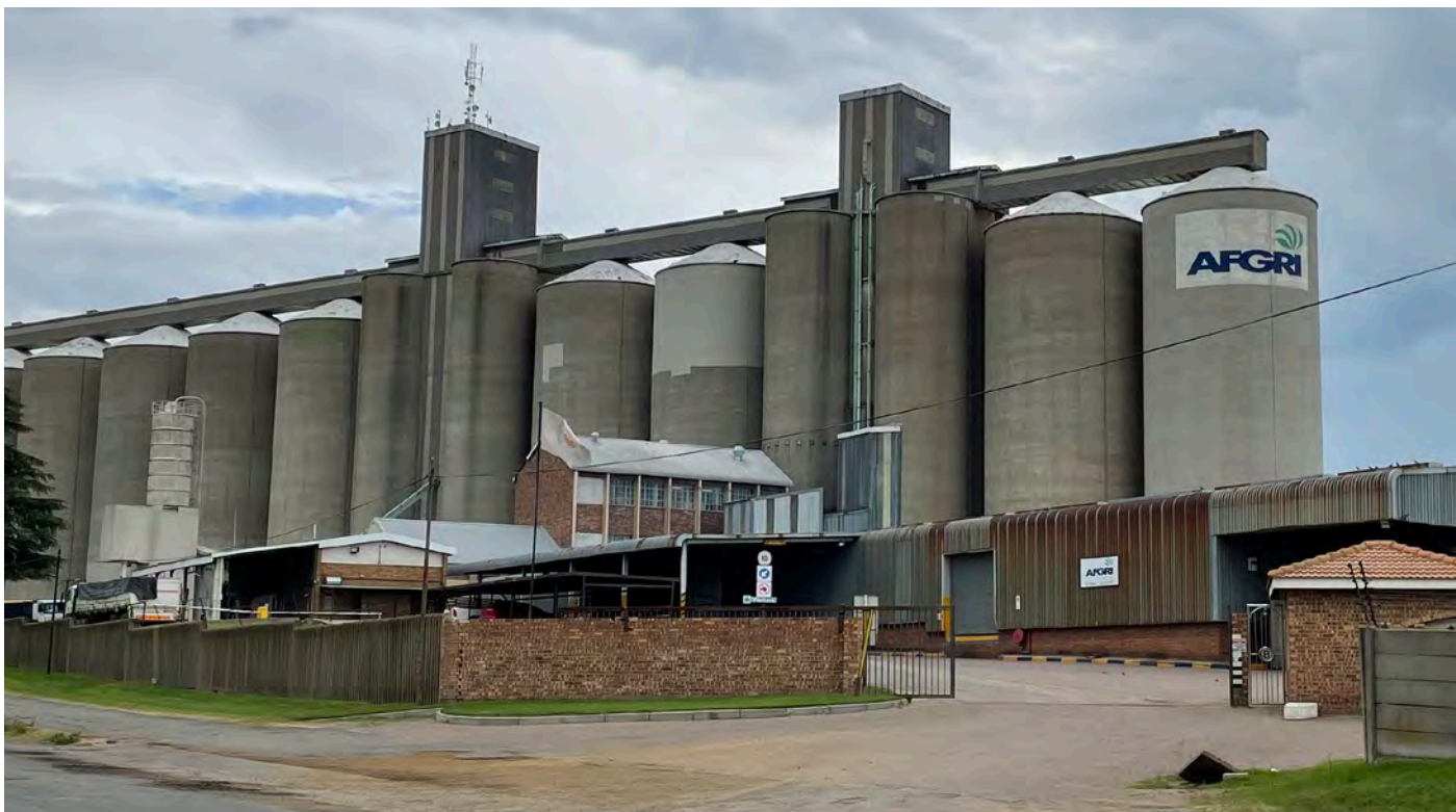
The grain silos of AFGRI in Ermelo, Mpumalanga. Grain silos are valued using the income capitalisation method of valuation, which means the income is calculated by analysing long-term occupancy figures and applying market-related tariffs.
