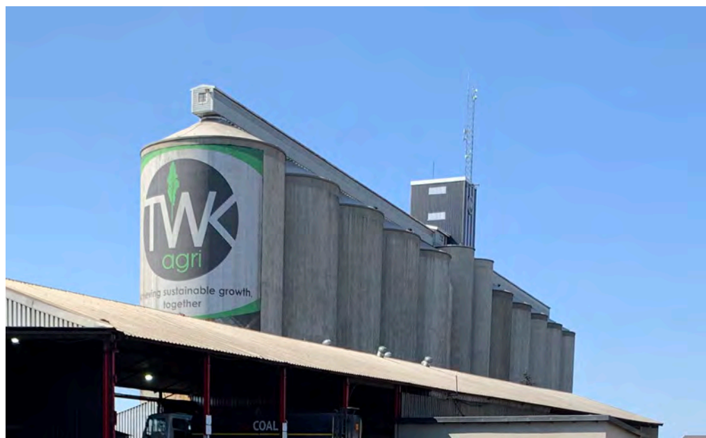
TWK's grain silos in Panbult, Mpumalanga. A grain silo is essentially an income-producing property and because the tenant is harvesting grain, the income will fluctuate.
