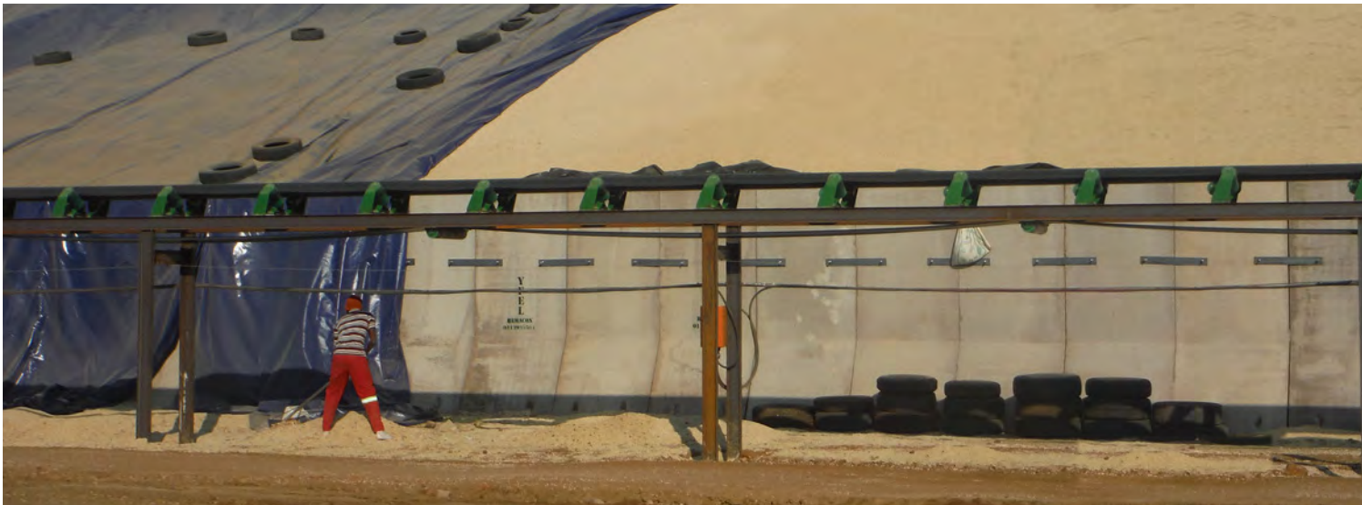
Yfel barriers at one of GWK's bunkers.
